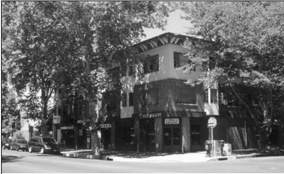
Housing over retail shops
